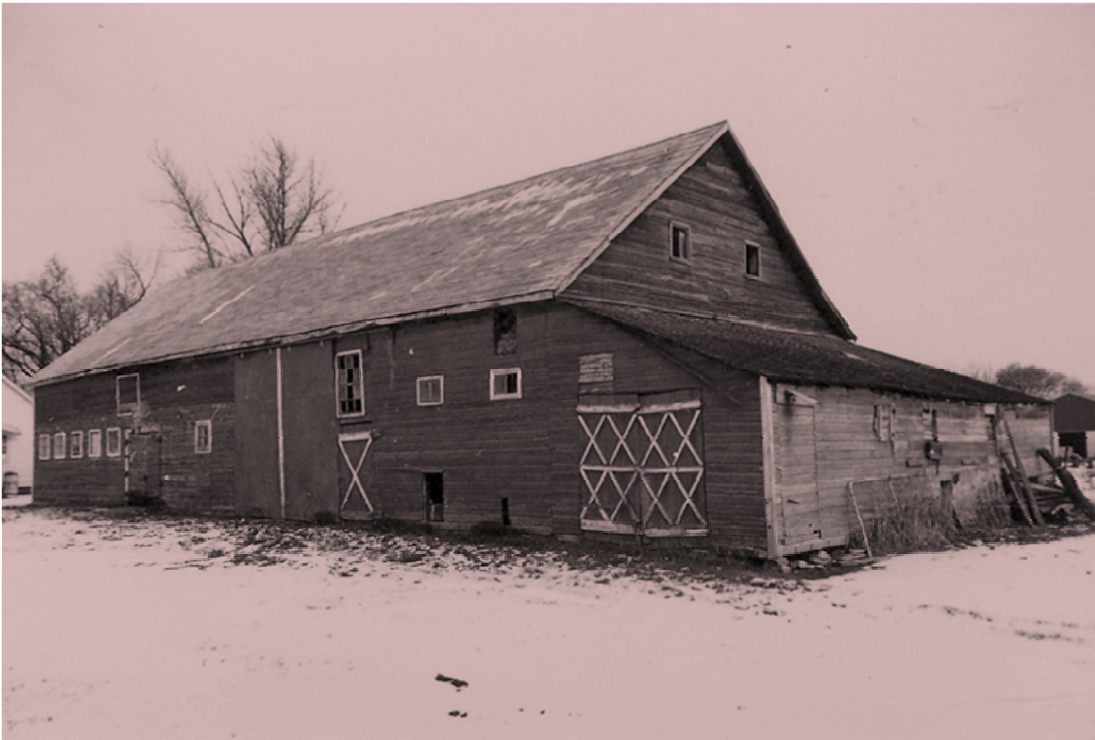
Figure 37 P.A. Rempel barn, Village of Neuenburg. Although not part of the traditional barn design, a rear "Sheua" section was often added to the barns in the MSTW district.
