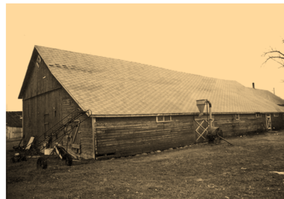
Figure 36 Hiede barn, Village of Hochfeld. A number of barns in the MSTW villages had wide "Owesied" sections, part of which acted as a second stable area.
