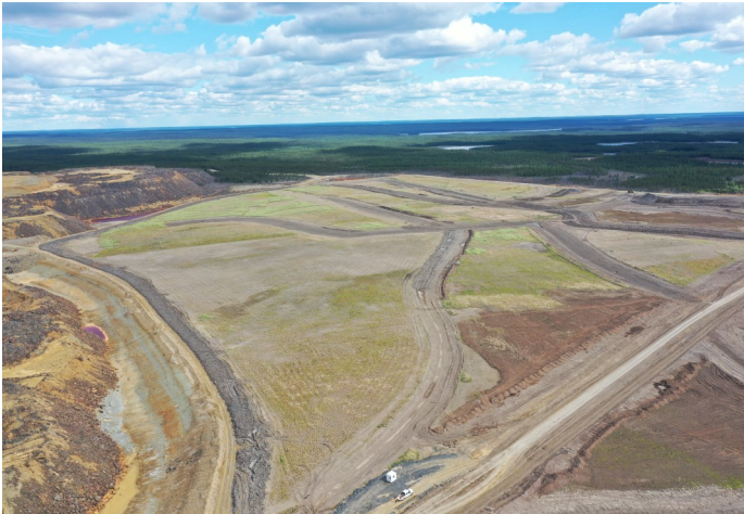
Tailings Management Area 1 - Northwest Corner of the Ruttan Mine Project site
