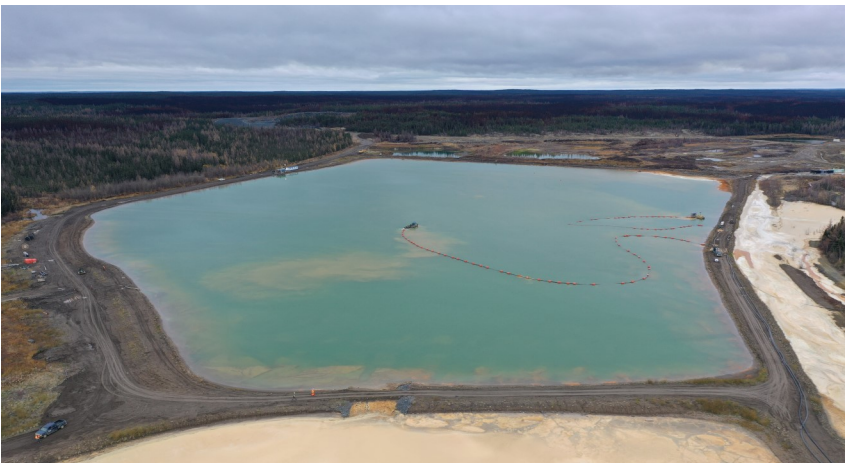
Settling Pond facing south east of the Ruttan Mine Project site
