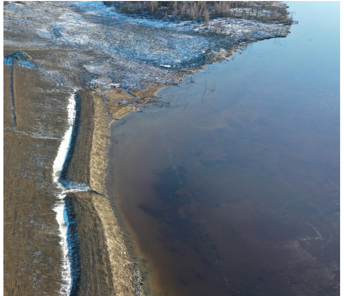
South End of West Dam
