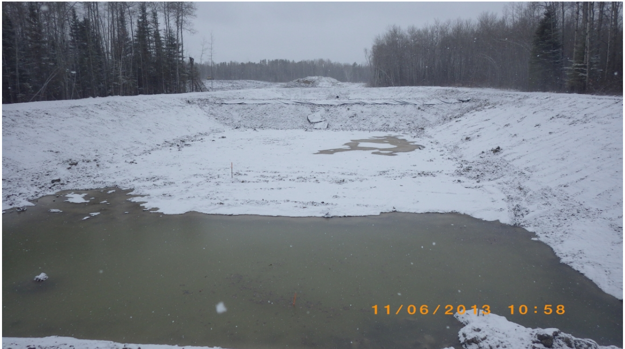
Photo 2 – North settling pond, southward view toward access road.
