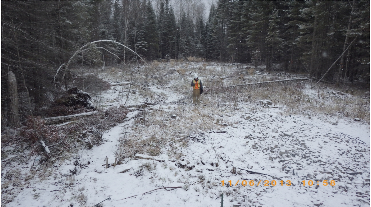
Photo 3 – Rock lined natural drainage swale north of the settling ponds.
