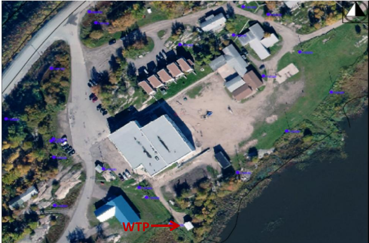
Figure 1. WTP Proposed Site
