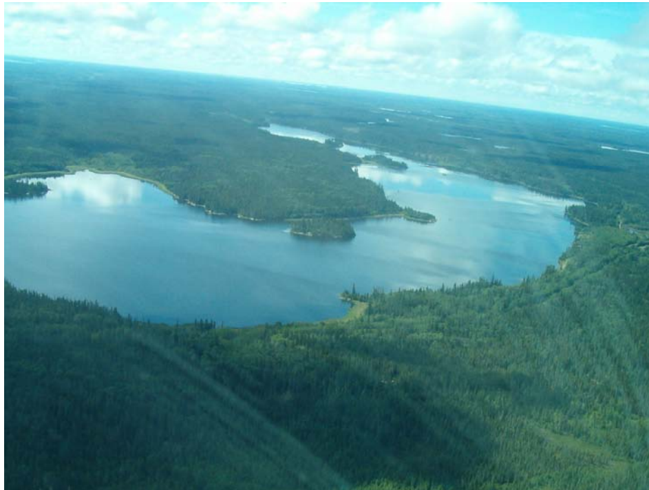
Photo 6: Anderson Tailings Impoundment Area (TIA)
