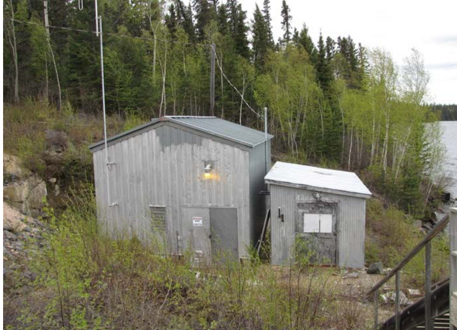
Photo 5: Snow Lake Pumphouse
