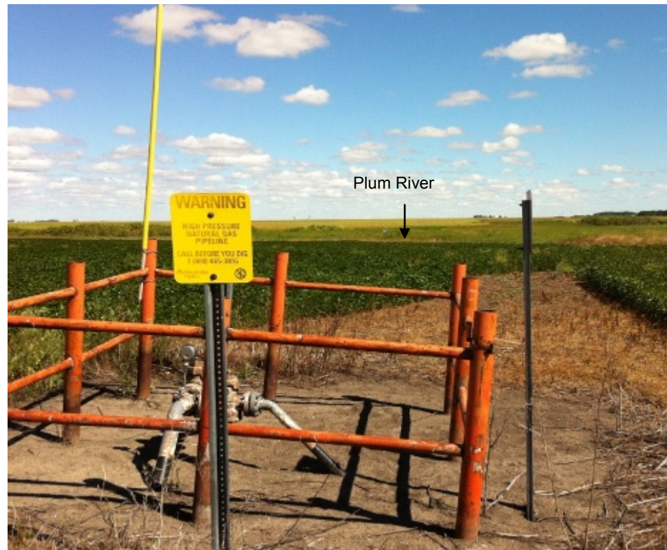
Photo 4: View facing north of the existing above grade valve assembly and Project area located on the south side of the Plum River. Manitoba Hydro file photo, July 27, 2012.
