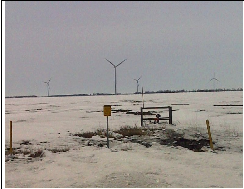
Photo 1: View facing south of the existing above grade valve assembly, existing RoW and Project area at the south side of PR201. April 20, 2013.
