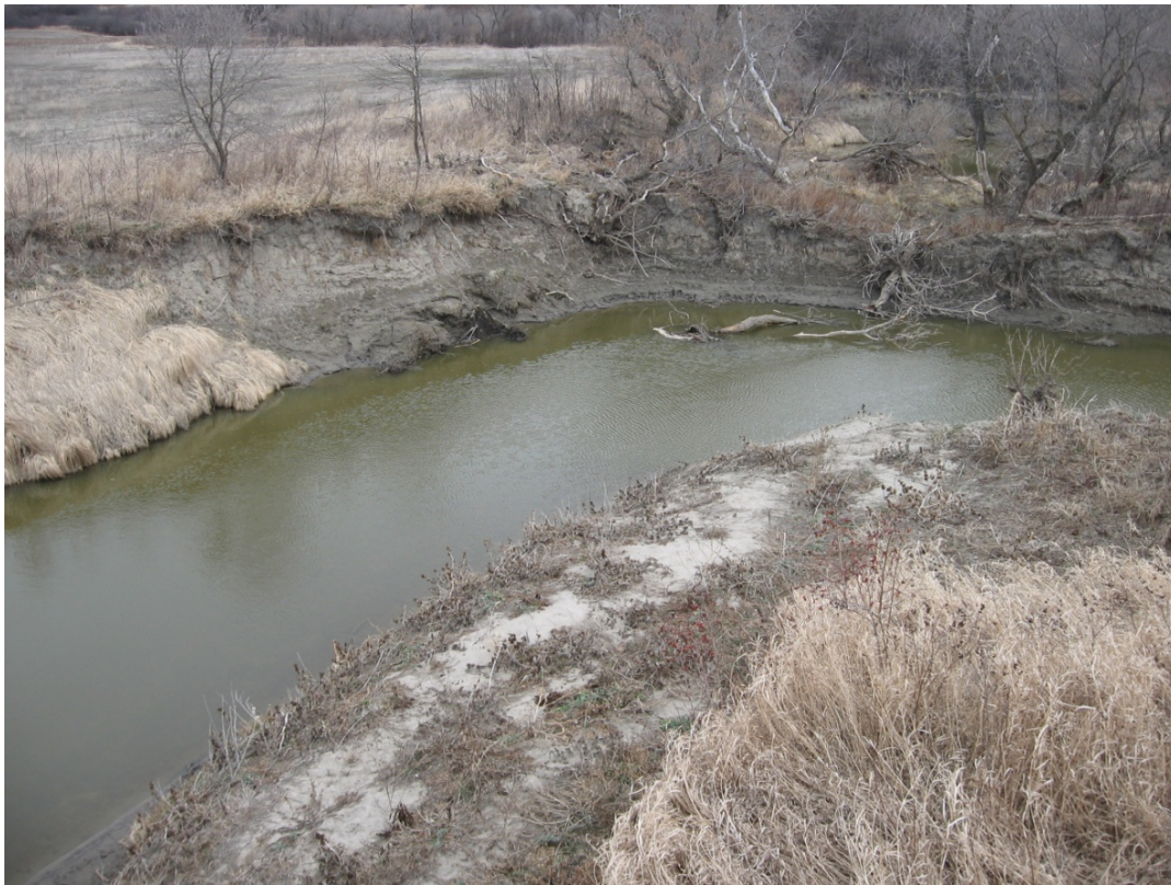
FIGURE 4.3 BRIERWOOD CREEK FOURTH ORDER DRAIN - APRIL 2, 2012
