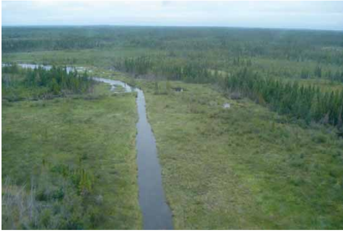
Photo 1. Looking towards crossing Site 23 from Butnau dyke.
