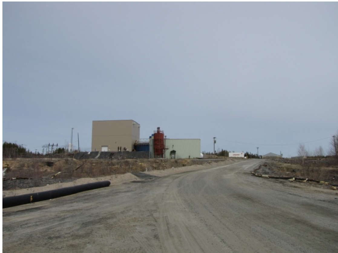
Chisel Water Treatment Plant
