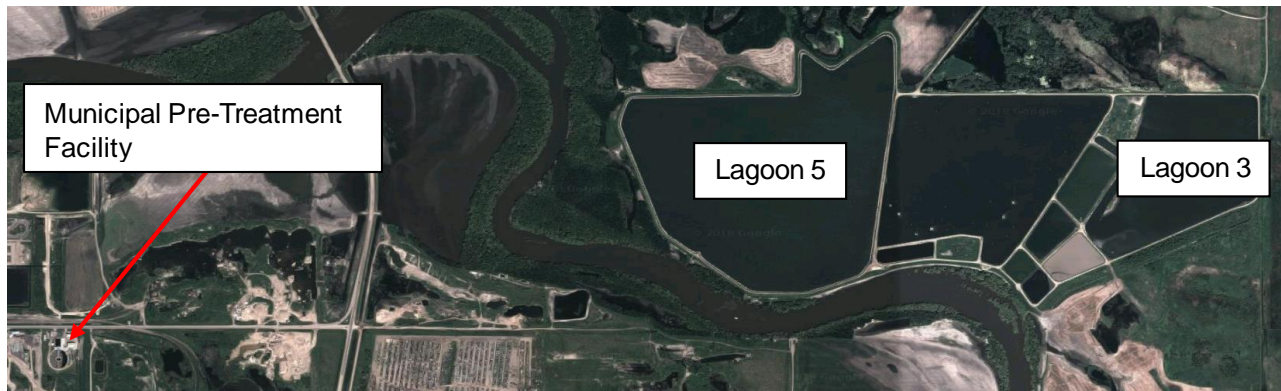
Figure 5-1: Municipal Pre-Treatment Facility
