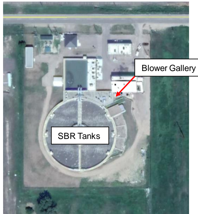
Figure 2-1: Municipal Pre-Treatment Facility
