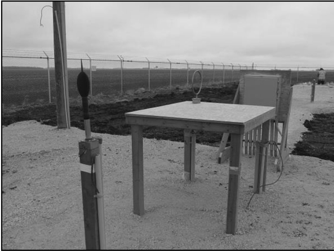
Figure 23: Noise meter microphone (foreground) and radio noise loop antenna (background on far corner of table) on south edge of row at southeast corner of main station.
