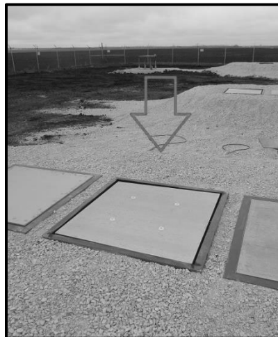
Figure 27: Wilson plate secured in gravel mound.
