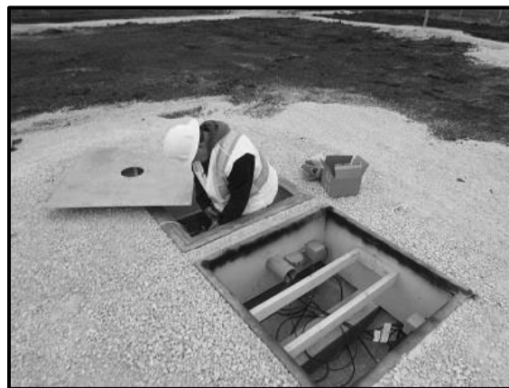
Figure 36: Installation of electronics for E-Field Mill.
