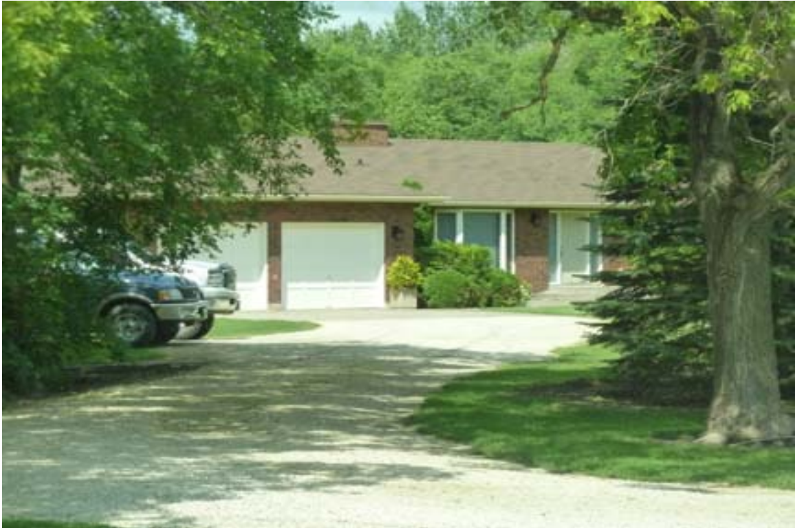
Photograph House at NE7-7-4E1 – R12
