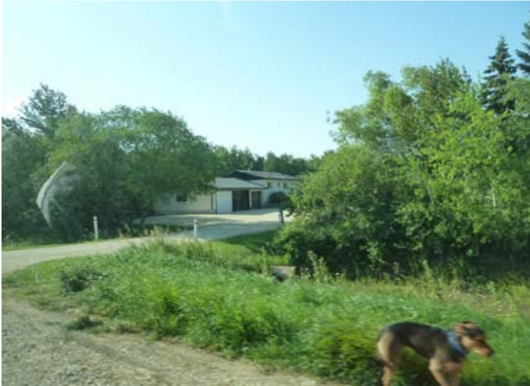
Photograph House at NE21-10-5E1 – R2
