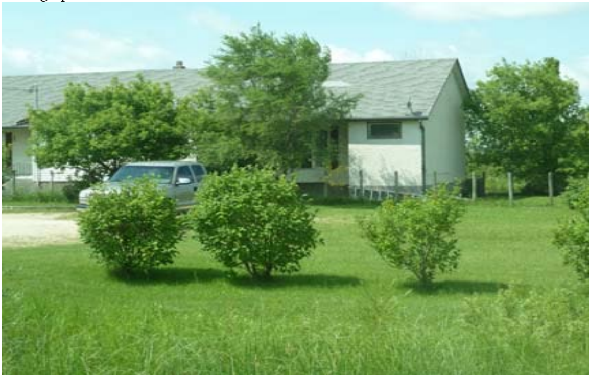
Photograph House at NE8-7-4E1 – R11
