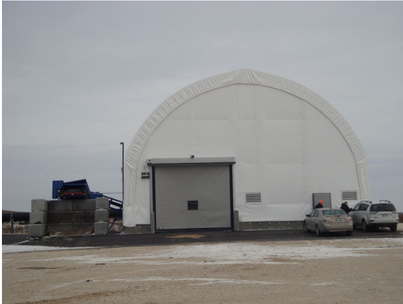
Figure 7 Biosolids Storage Building
