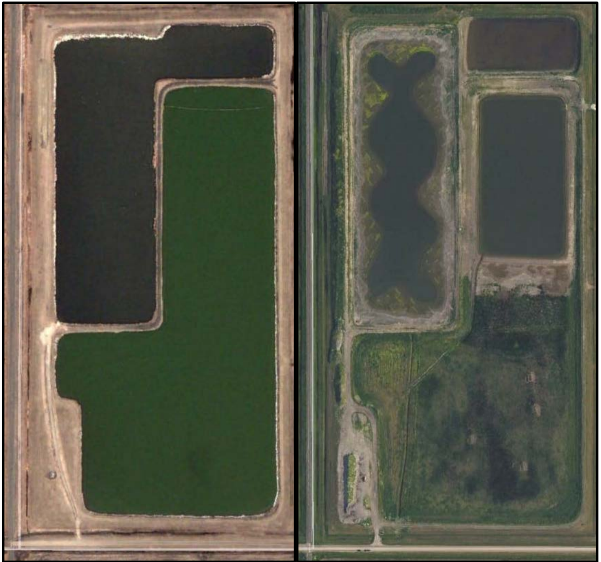
Figure 2. Niverville lagoon on SW 30-7-4 EPM during operation in 2002 (left; Image courtesy of Google Earth) and in 2013 after redesign for the Niverville Lagoon Bioremediation Project (right; Image courtesy of Google Earth.)
