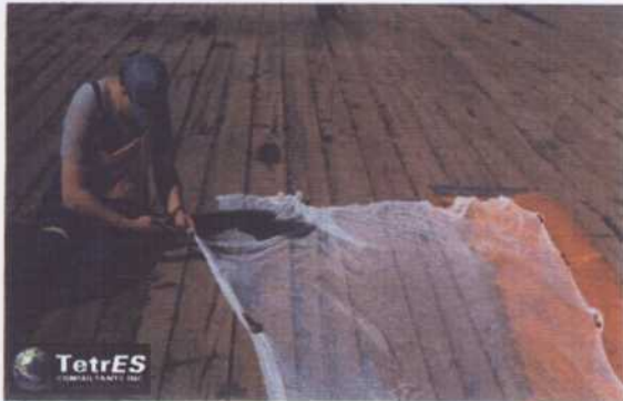
Figure 3: Metal weights are secured to the bottom of the mesh net to keep the curtain in the desired position as it hangs suspended from the floating boom.
