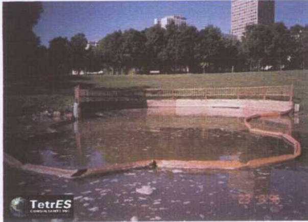
Figure 8: The Combined Sewer Outfall at Juba Park serves the Bannatyne Sewer District. The configuration of this outfall makes it an ideal location for boom installation.
