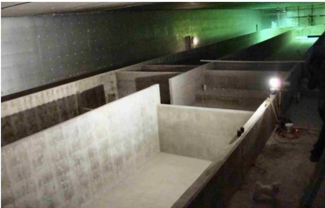
Figure 12: View of the completed concrete walls of the water reconditioning system.
